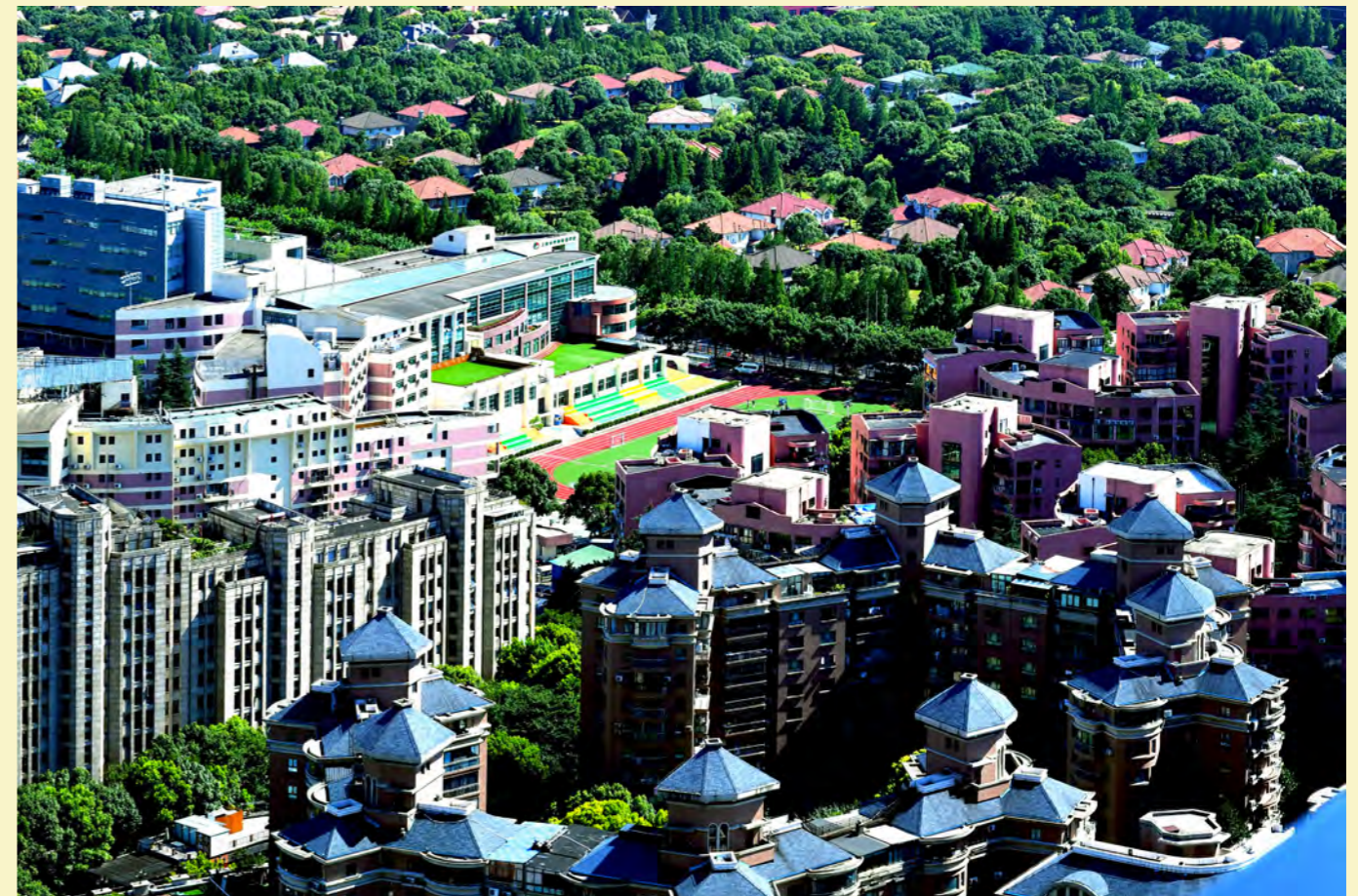
Biyun international community in Jinqiao, 2018. It has transformed from a supportive living community for the industrial companies in Jinqiao into an international community integrated with the whole city. (Photo / MAO Zhengyuan, Image Source / The Eyes of Pudong, Documentary Photography)
